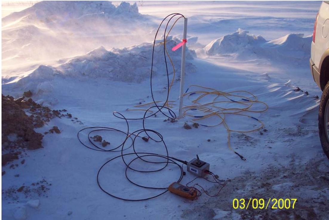
Figure 6: Thermistor and Bandgap-Based Digital Cables Installed in Nome Test Boring
