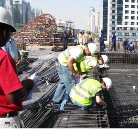
student interns are tying rebars at a construction site.
