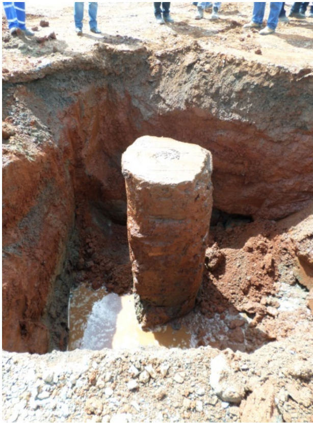
Fig.8 photo. Excavated DSM-column
