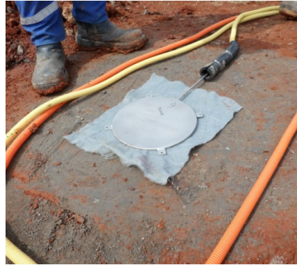
Fig.10 photo. Load cell installed on top of a column
