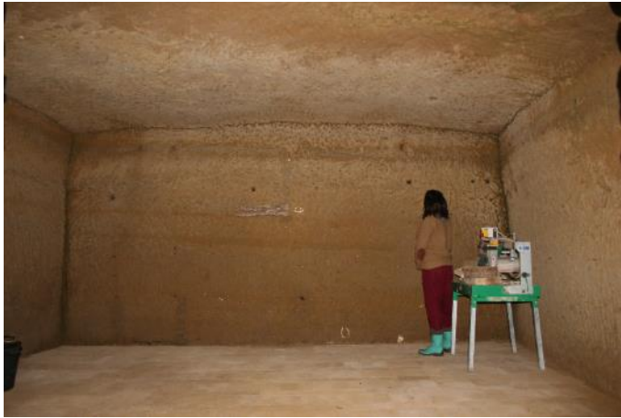
AT Cave excavated in unsaturated silty sand
