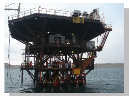
Offshore structure, Talara, Peru
