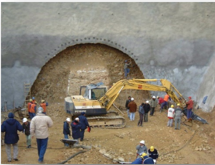
Cerrillos tunnel, Bolivia
