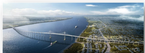
Demerara Bridge, Georgetown, Guyana
