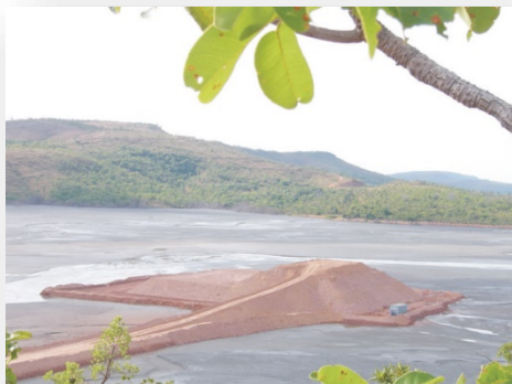
Trial Embankment on tailings
