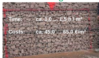
b. Finalised repair
