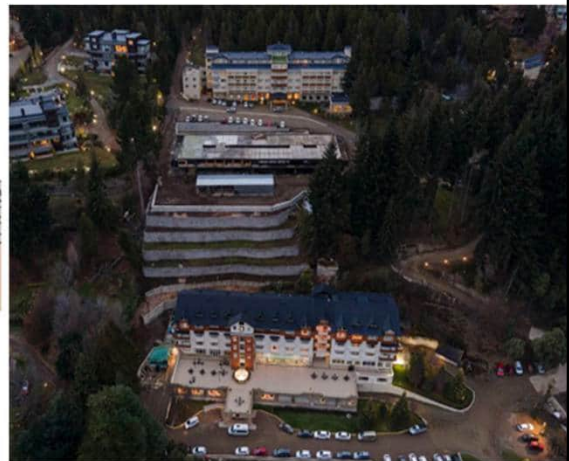
Mendiz, De Loyola, Dal Farra & Ardila Montilla (2024). Mechanically Stabilized Earth (MSE) retaining wall at Hotel in Bariloche City .
