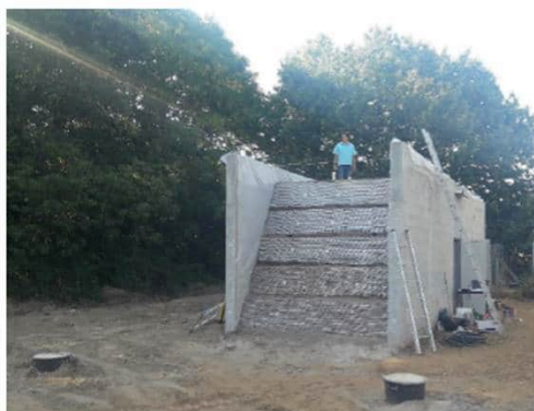
End of construction
