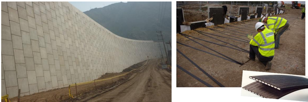
Figure 10: Typical MSE front facing view and reinforcement installation.
