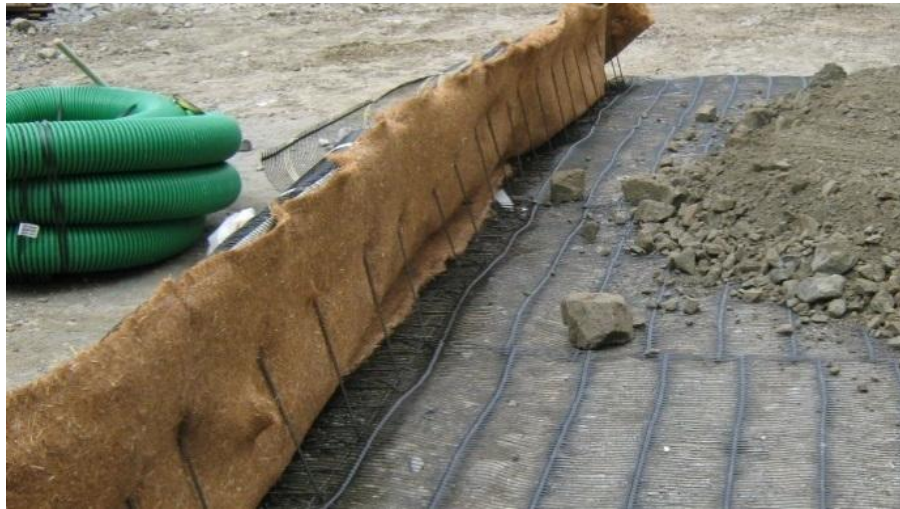
Figure 3 Installation: from the left, steel mesh formwork, geogrid, straw mat, and fill material.
