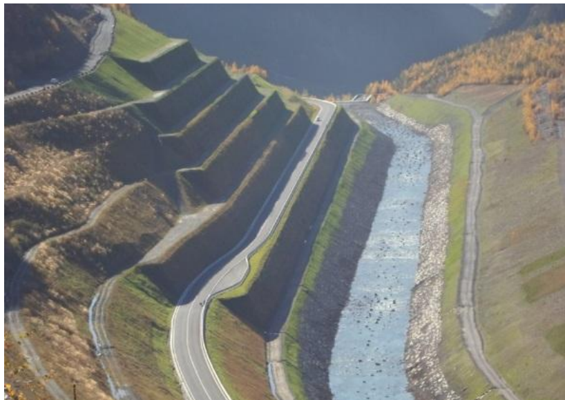
Figure 4 The finished job.
