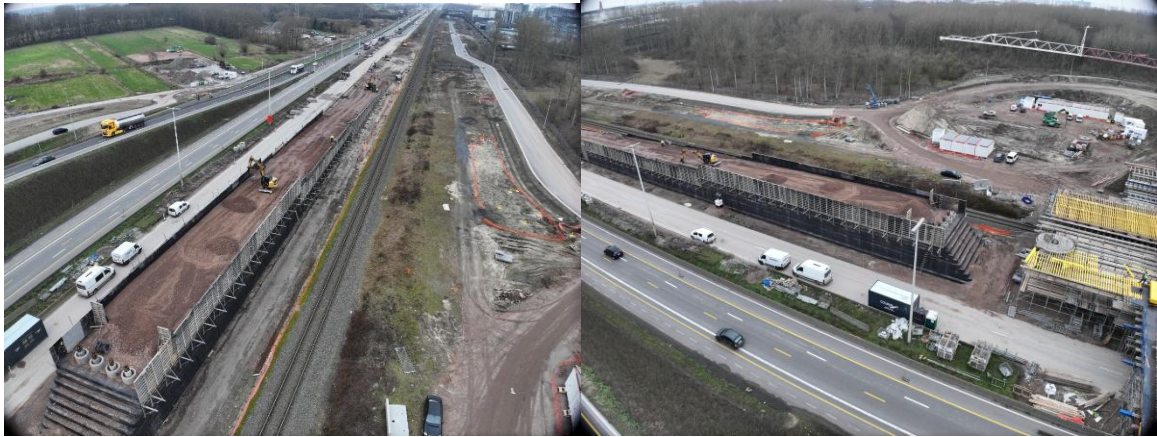
Figure 1: Reinforced fill structure build with recycled aggregates as fill material in the scope of the works on the R4 ring road in Ghent (Belgium)
