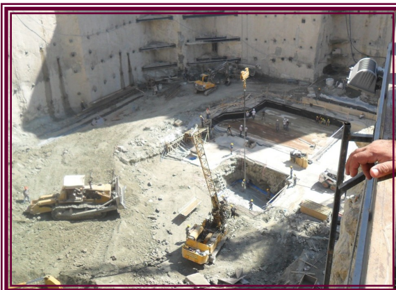
Below: Excavation site
