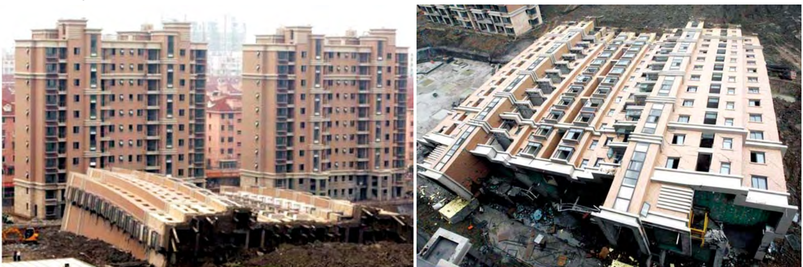
Figure 1: Two views of a toppled 13-storey apartment building that buried one worker in Shanghai on 27th June 09. Photo: Reuters
