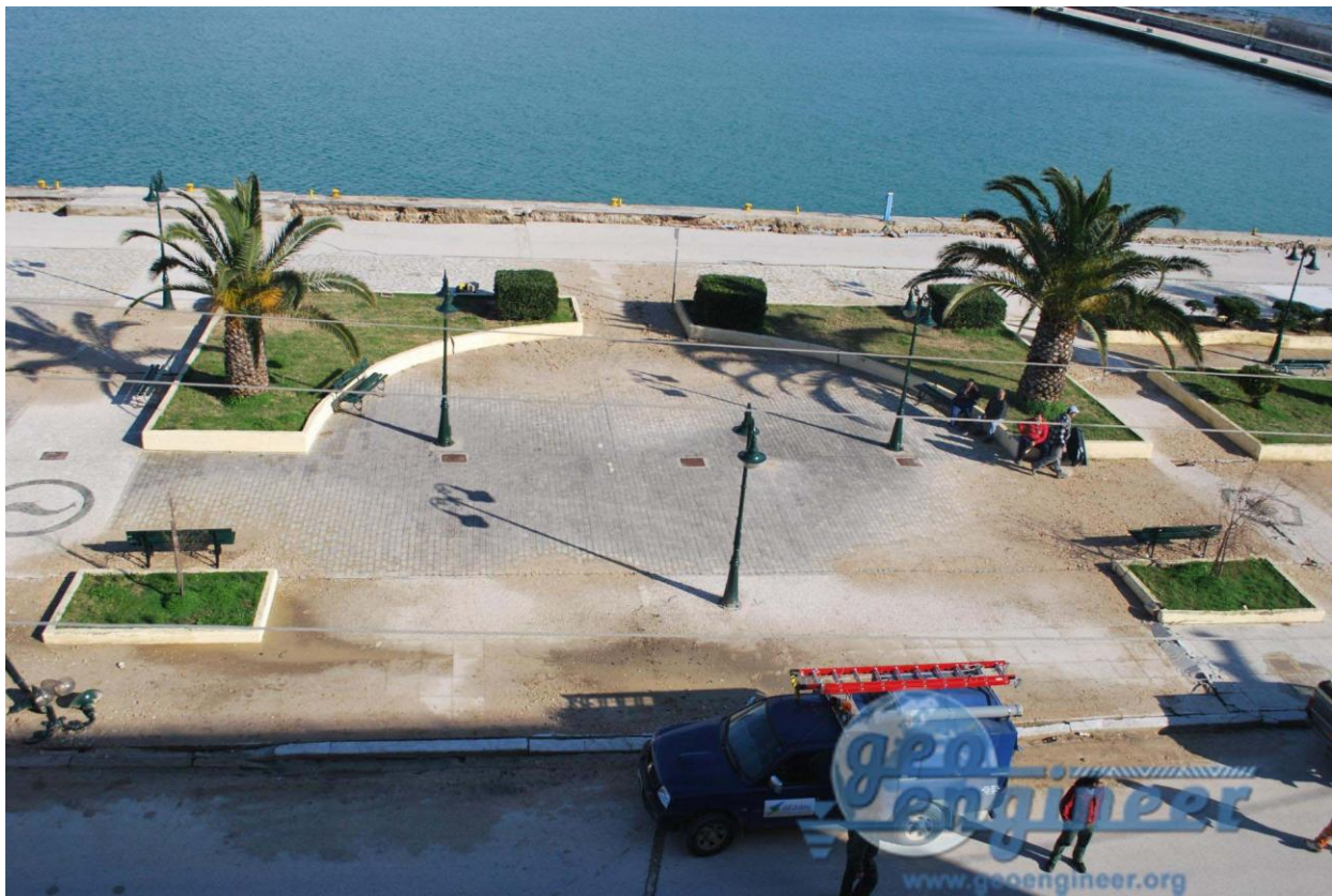
Picture 12: Indications of liquefaction (Corner of Laskaratou & Skarlatou, Lixouri).
