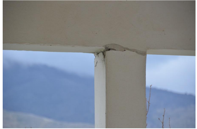
Photo 4. Damage to column-beam joints of the building of Photo 3 .
