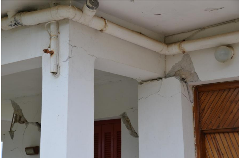
Photo 4. Damage to column-beam joints of the building of Photo 3 .
