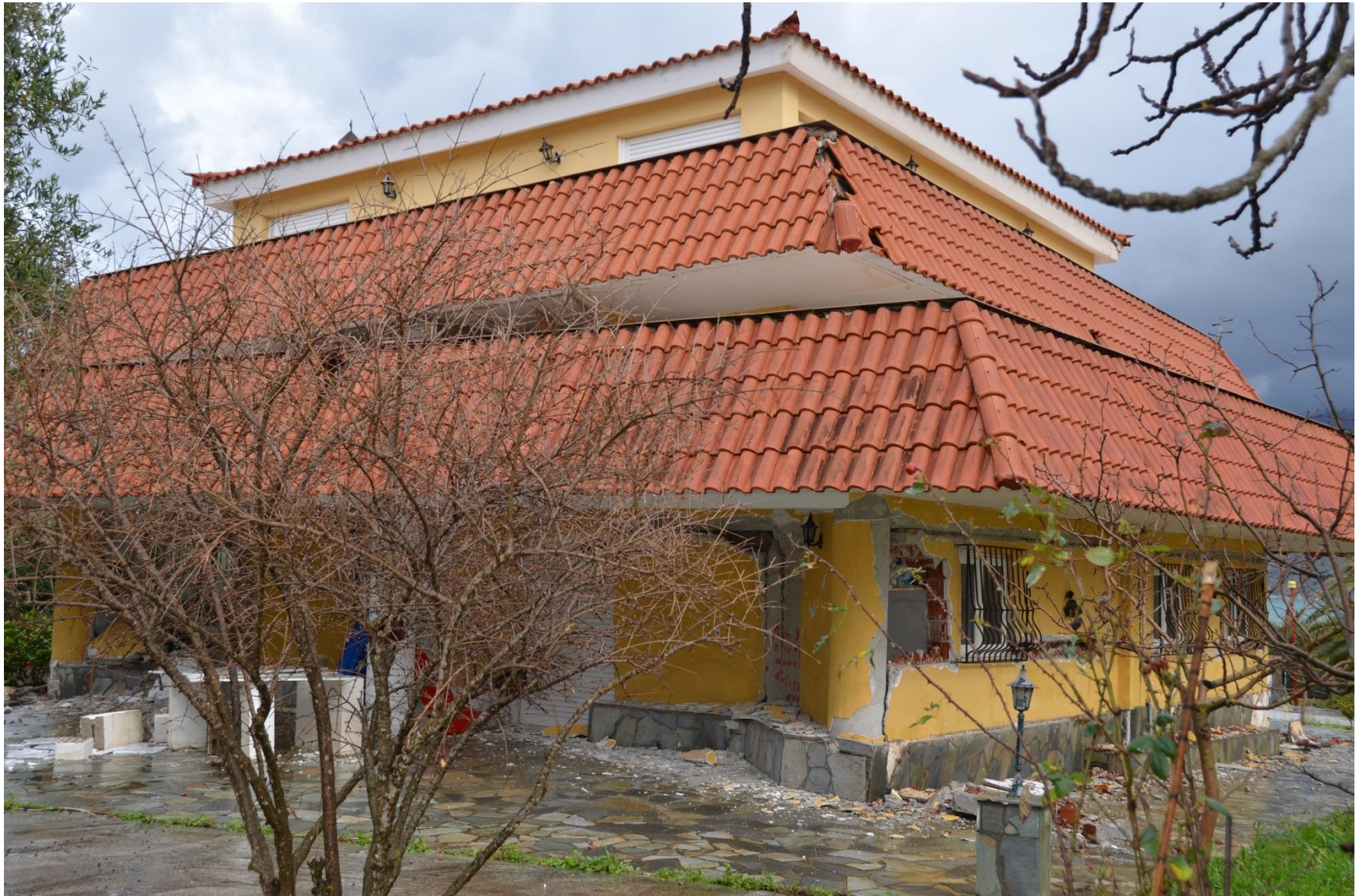
Photo 1. Total collapse of the second floor of a three-story RC building at Leivadi. The building had a 'pagoda' shape with reduced plan dimensions from floor to floor (the perimeter columns of each floor were not continuing to the upper floor).
