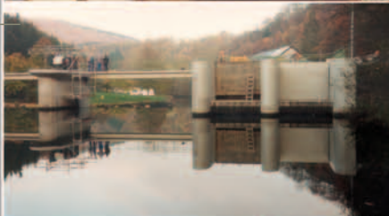
Dam on the Sure River (Luxembourg) Diagnostic and safety study
