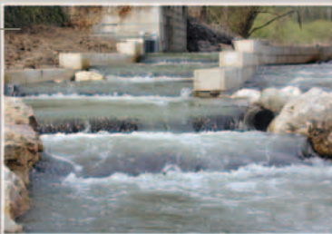
Fish ladder on the Allondon River (Switzerland) Design and project management
