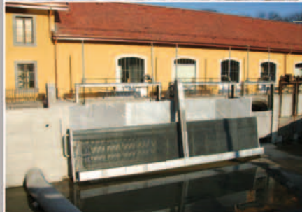
Vessy hydropower plant (Switzerland) Design and project management
