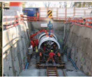
■ Choully sewage transfer tunnel, St Genis-Pouilly (France) Design and project management
