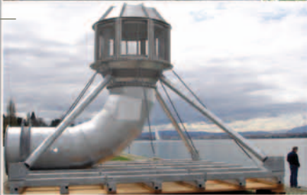
Offshore water intake in lake Geneva (Switzerland) Design and project management
