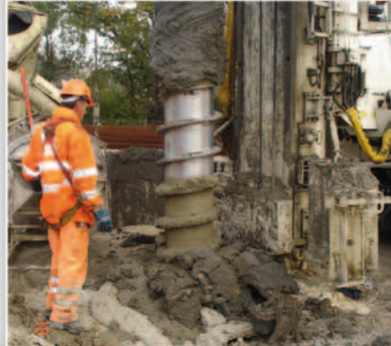
■ Bored piles with a hollow auger
