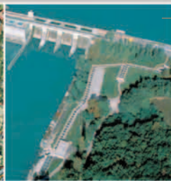
Fish ladder at Verbois dam (Switzerland) Design and project management
