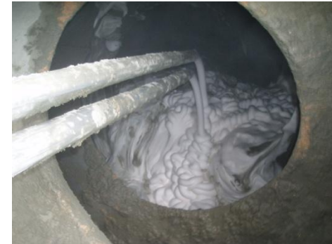
Foam batching in mixer truck
