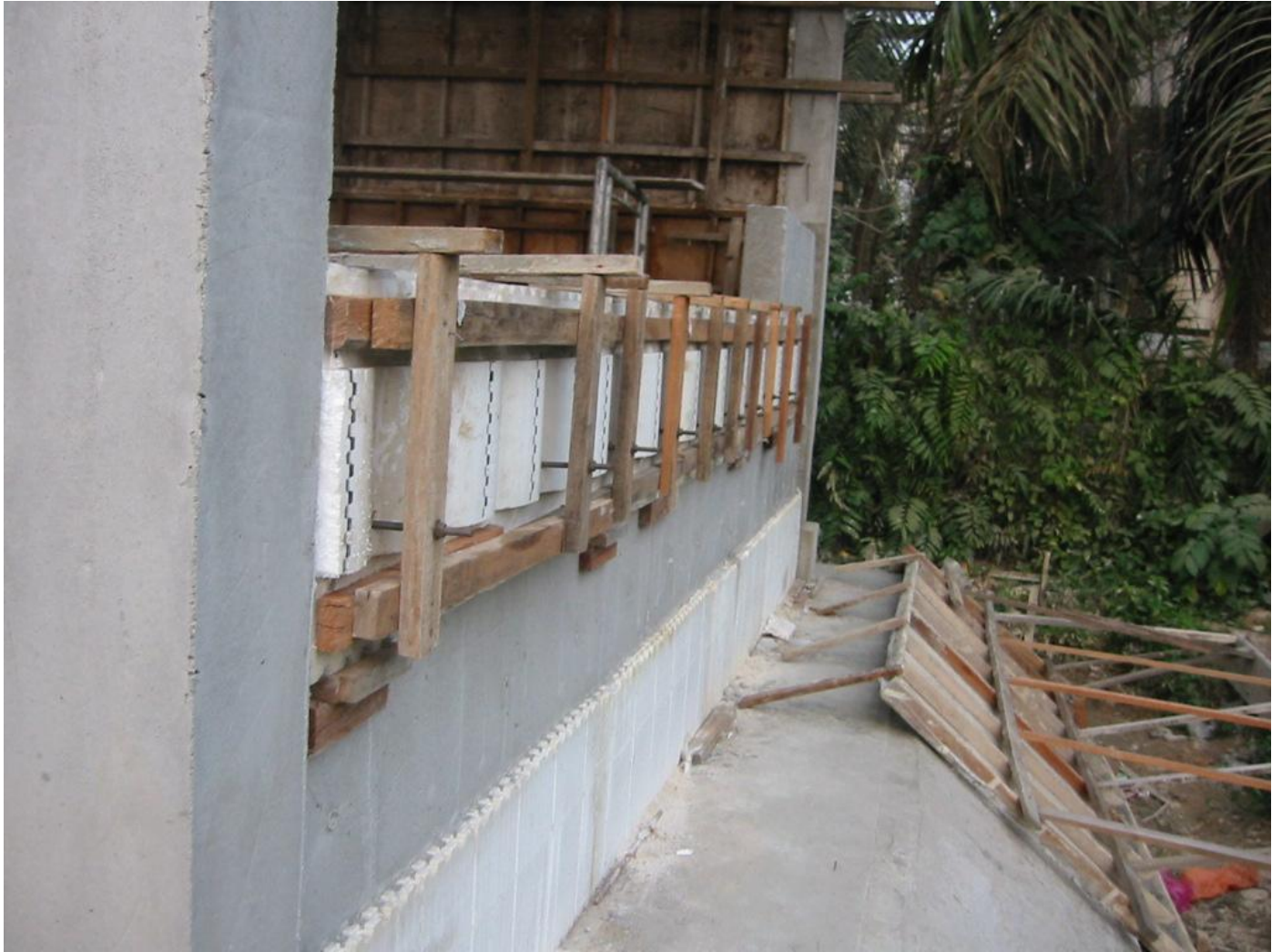
KUiK formwork with profiled expanded polystyrene panels
