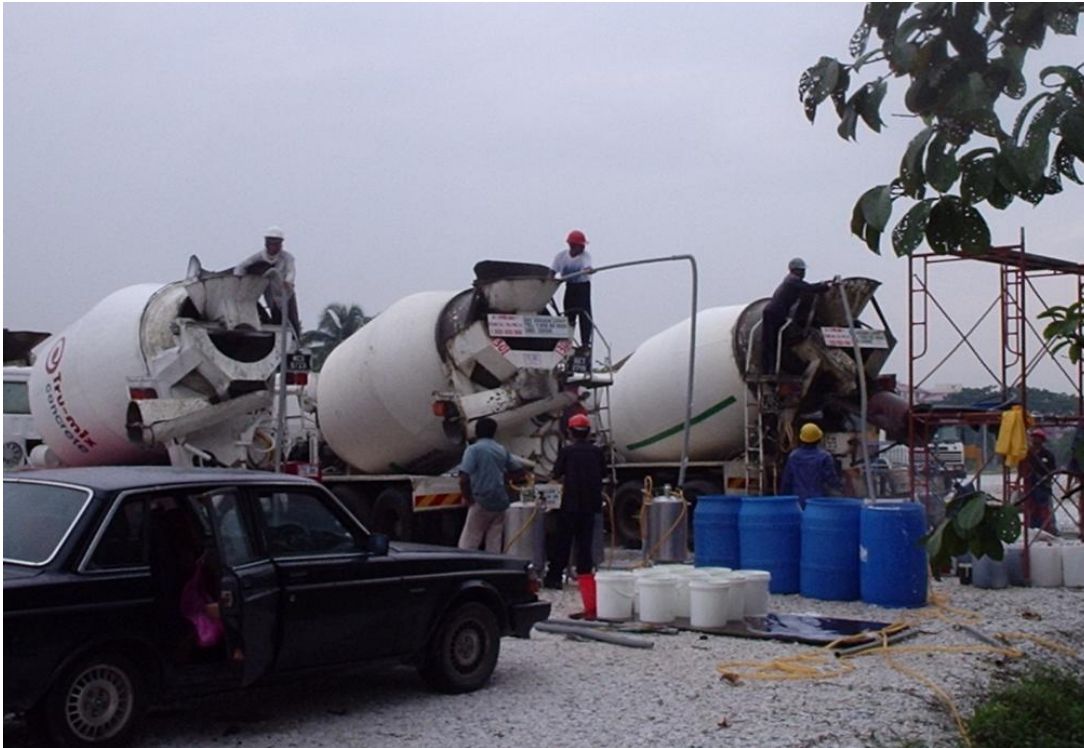
On-site production of KUIKcrete
