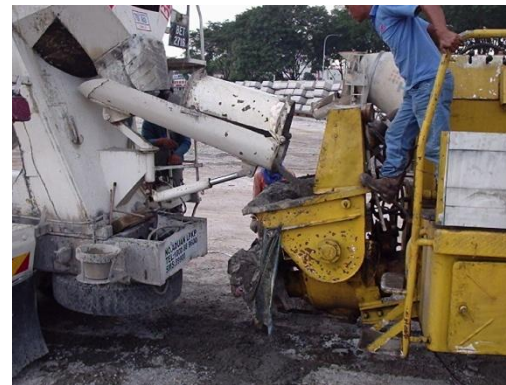
Mixer truck to concrete pump
