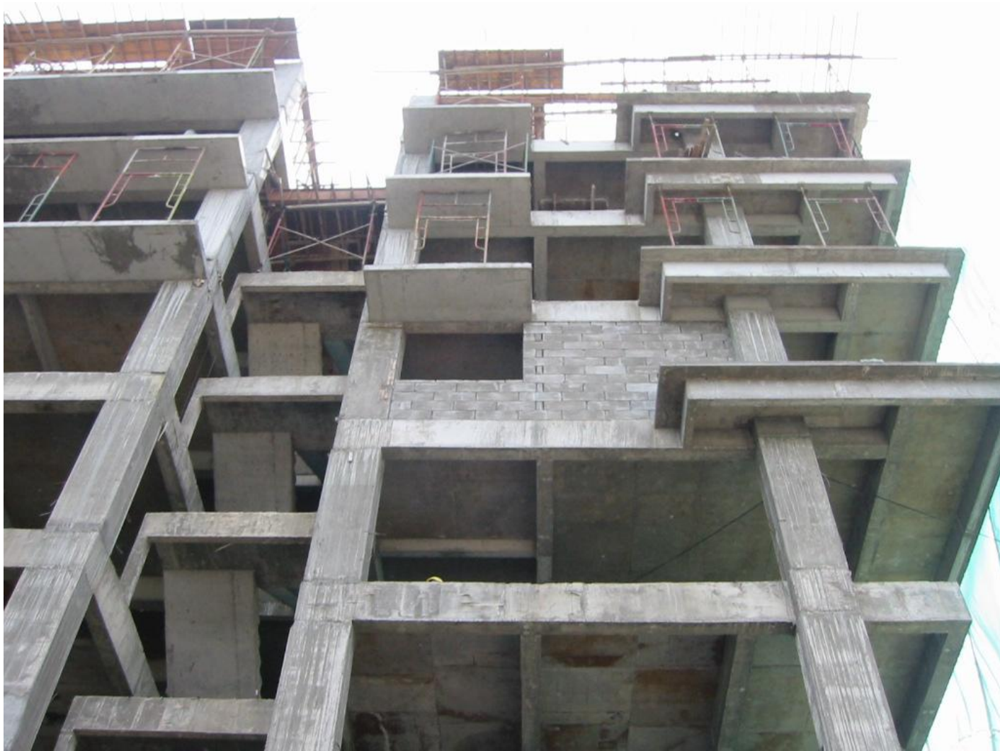
KUikwall in highrise construction
