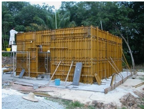
Casting of foamed concrete into system formwork
