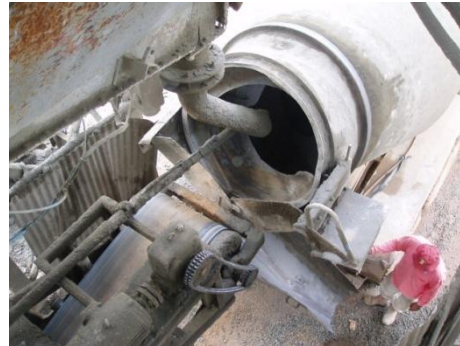
Cement & sand is batch in mixer truck
