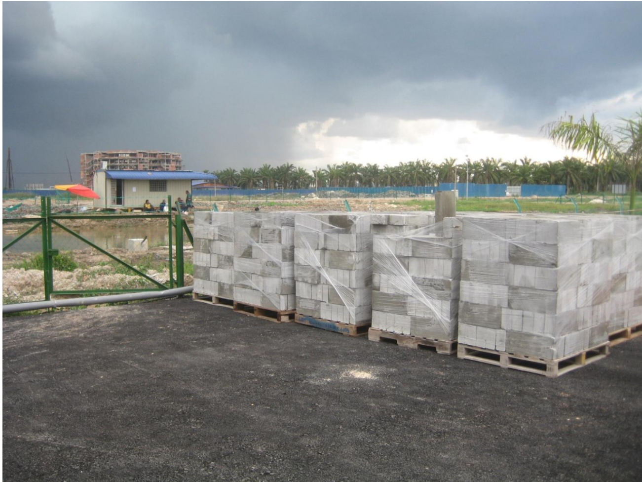
KUIK Block for soft soil subbase system
