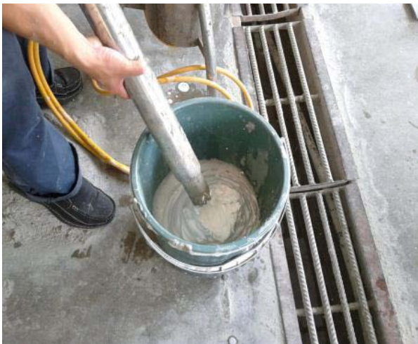
Figure 5. Foamed concrete for casting
